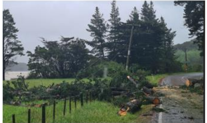
Photograph 4: Line damage in Tirioto caused by trees outside the fall zone in November 2022
