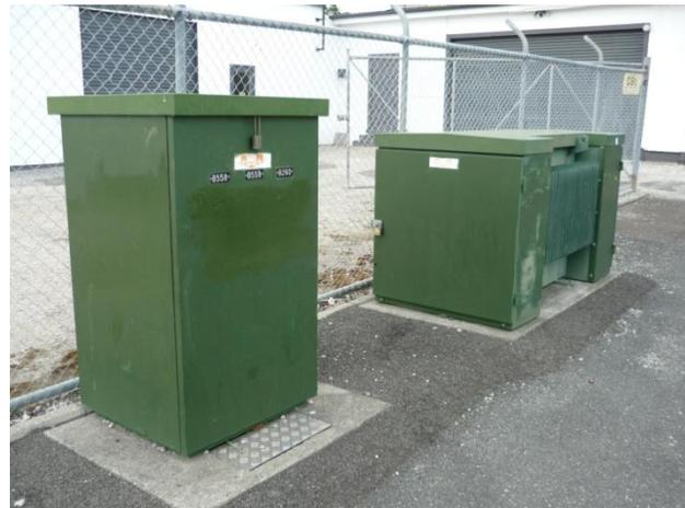
The distribution switchgear associated with the underground distribution network substations is predominantly ABB SD series Oil filled switchgear or ABB Safepus SF6 gas filled switchgear. Switchgear installations are pad mounted and either located adjacent to or a short distance away from the substation installations.
